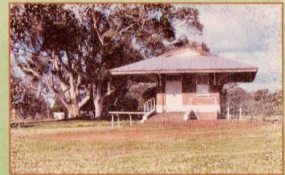
Darkan Railway Station
